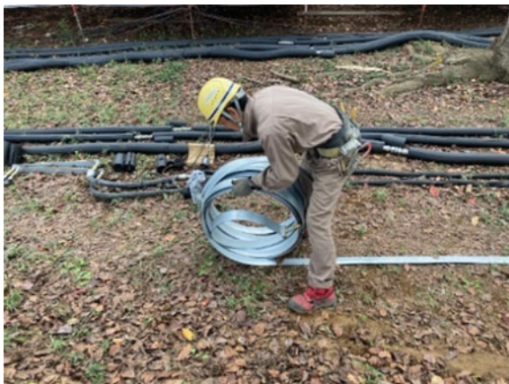
Fig. 15 Placing 50 m long freezing pipe
