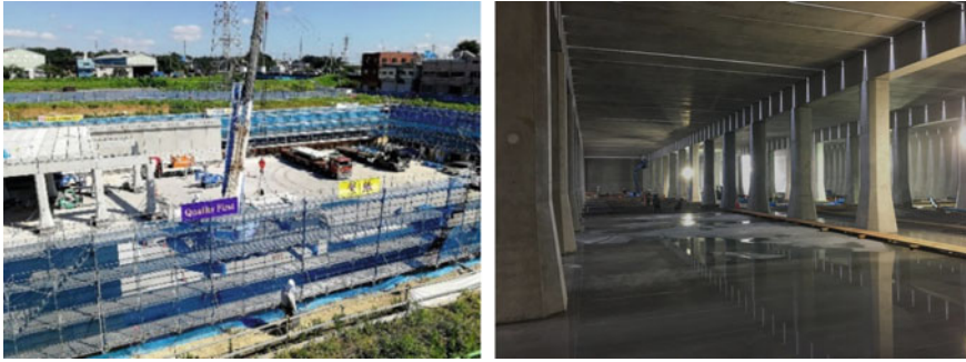
Picture 1 Underground reservoir under construction in 2019
