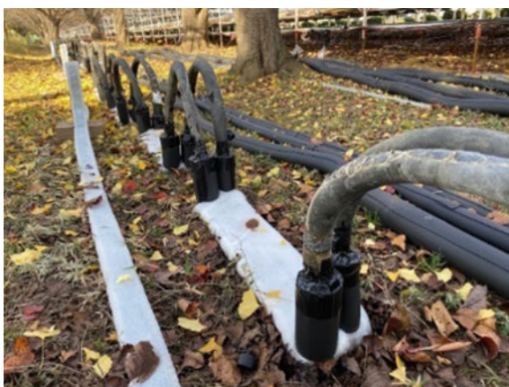
Fig. 17 Connecting freezing pipes
