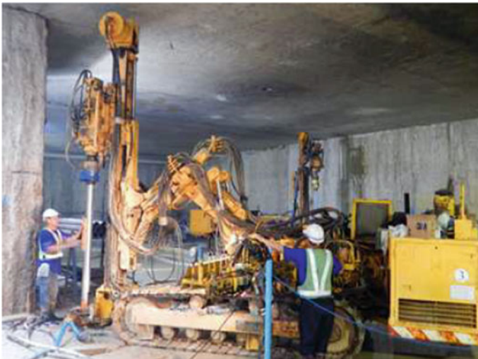
Fig. 8 Tube-A-Manchette (TAM) grouting operation at BS12 station box
