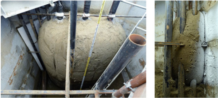
Fig. 11 Excavated frozen soils (left—guide pipe type, right—attached type)
