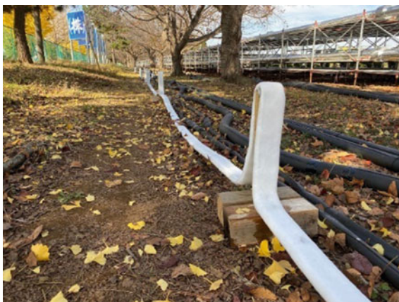
Fig. 16 Freezing pipe bent every 5 m
