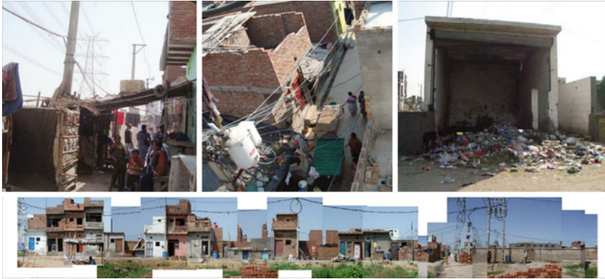
Fig. 6 Public interaction spaces (Left), poor structures (top center), and poor waste management on the site (Right). Building typologies that exist in the resettlement colony (bottom). Source [26]
