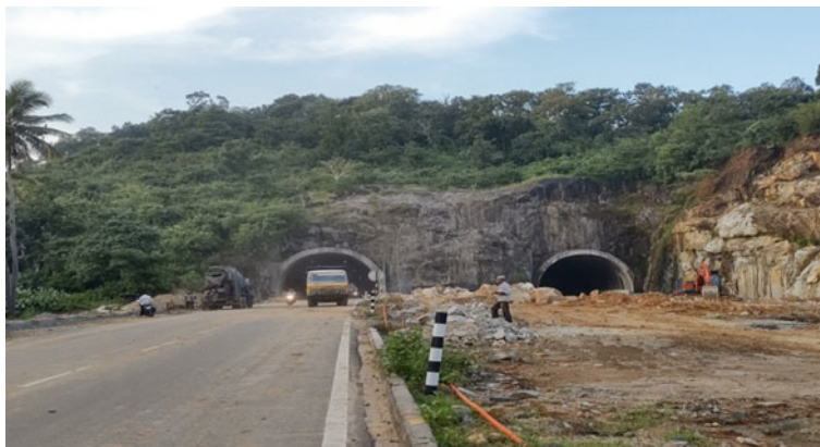
Fig. 1 Twin tunnel Karwar
