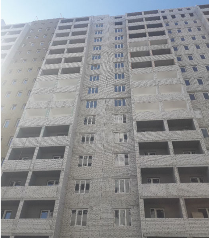
Fig. 9 Expansion joint at the final stage of construction
