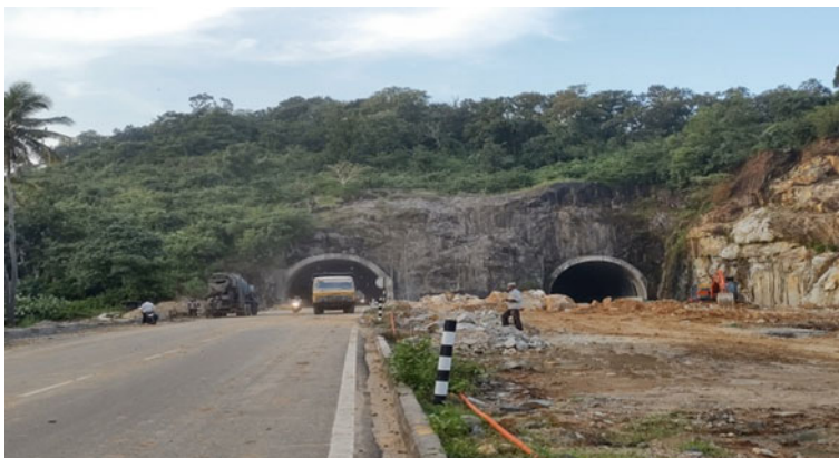
Fig. 1 Twin tunnel Karwar
