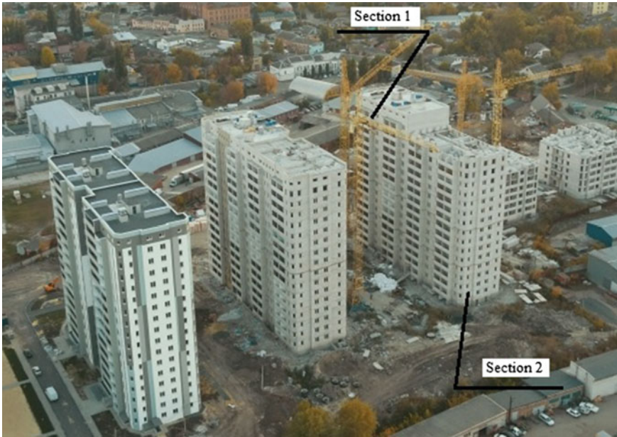
Fig. 1 Arrangement of the experimental building 7 (Sections 1 and 2) during erection
