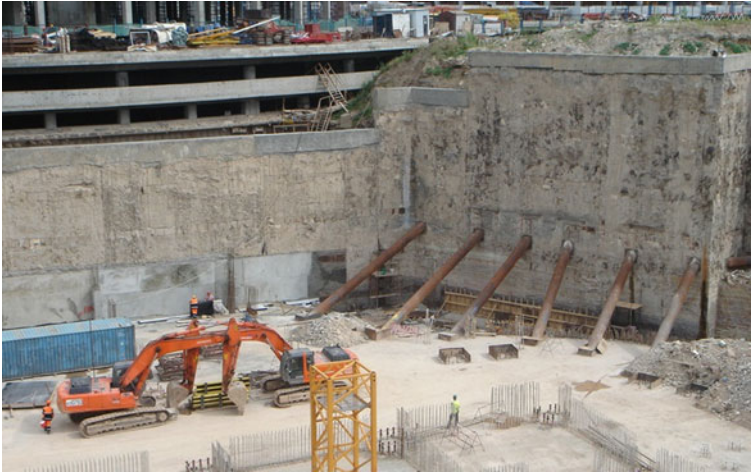
Fig. 1 Diaphragm wall. ( https://www.designingbuildings.co.uk/w/images/4/40/Diaphragmwall1.jpg ) [1]
