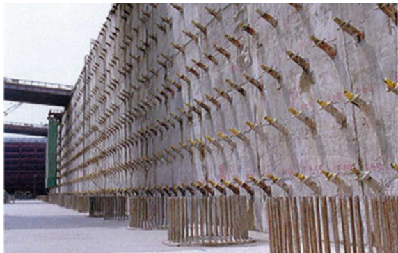
Fig. 6 Anchored diaphragm wall [20]
