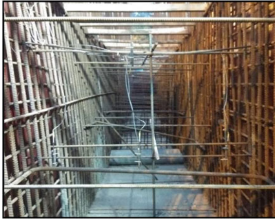
Fig. 11 Thermocouples fixed to rebar
