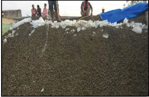
Fig. 5 Lowering aggregate temperature with ice
