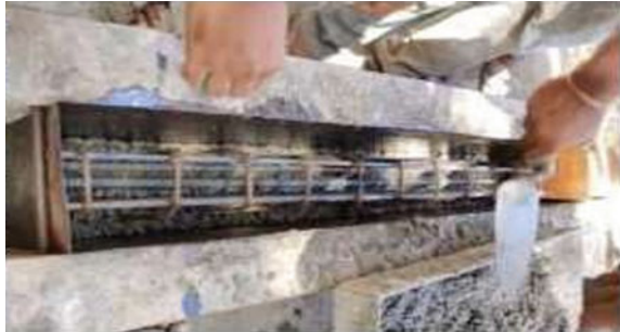
Fig. 5 Placing concrete in beam mould
