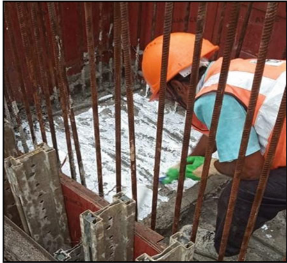
Fig. 7 Application of curing compound over concrete surface
