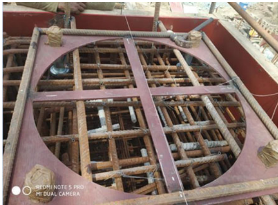
Fig. 15 Standard template in site to cast the pedestal
