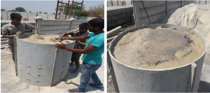
Fig. 5 Testing of soak pit
