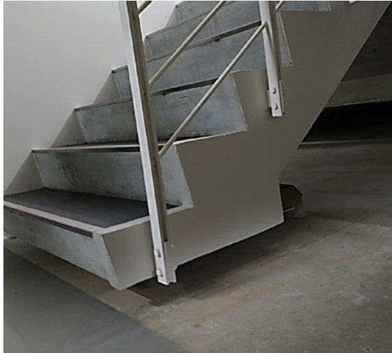
Fig. 10 Staircase flight joint between basement and ground
