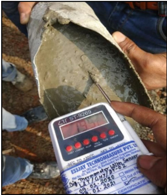
Fig. 6 Concrete temperature at pouring point < 25 °C
