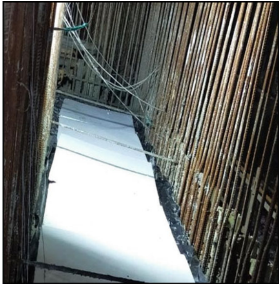
Fig. 8 Application of thermocol over LINAC slab
