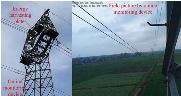
Fig. 11 Practical system in outdoor environment and the captured picture
