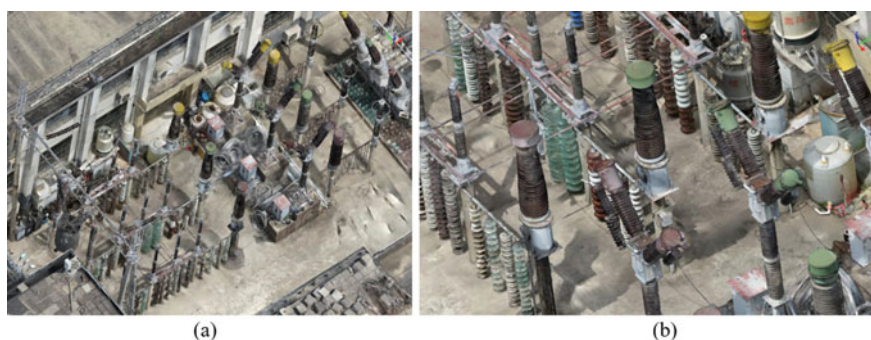
Fig. 5 The 3D model built by the method proposed in this paper. a 3D model of the substation; b 3D model of electrical equipment
