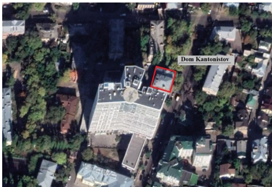
Fig. 2 Technogenic conditions of the site of the building—«House of Cantonists», Voronezh city
