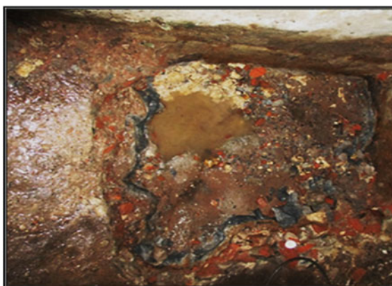
Fig. 3 Technogenic «top water» on the ground floor of the building «House of Cantonists»
