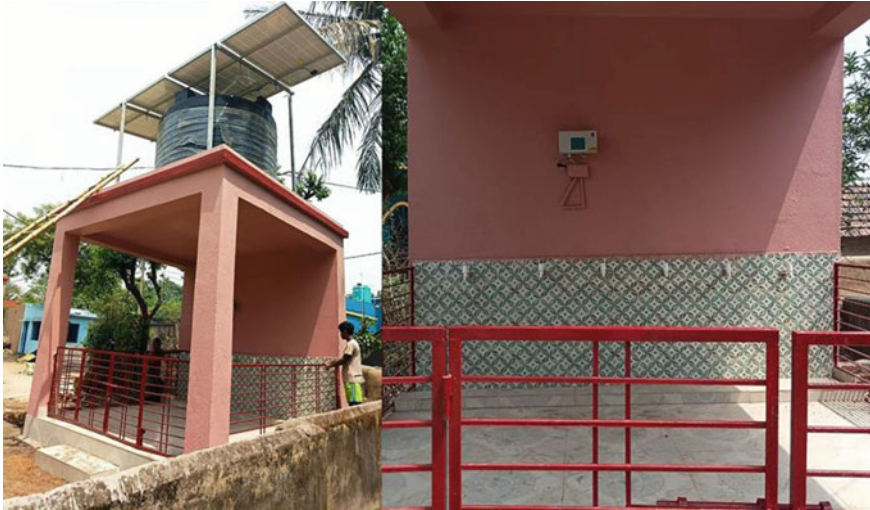
Fig. 2 Existing drinking water system at the proposed location. (Image source: Damodar Valley Corporation, India)
