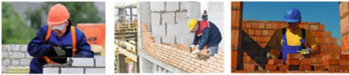
(a). Scene images of masonry work
