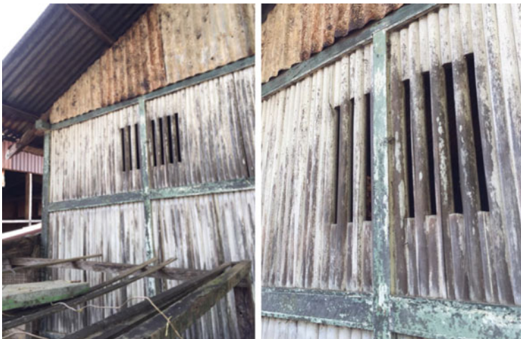
Fig. 3 Variation of ventilation in the walls of Rumah Gaba-Gaba in Merauke
