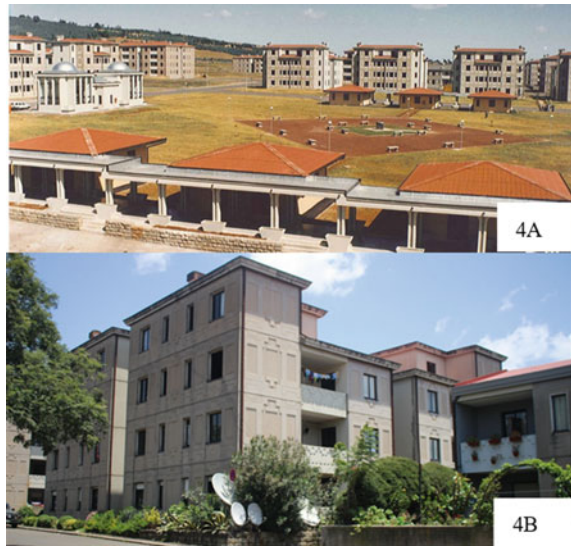
Fig. 4 CMC apartment buildings. Source CMC and Author
