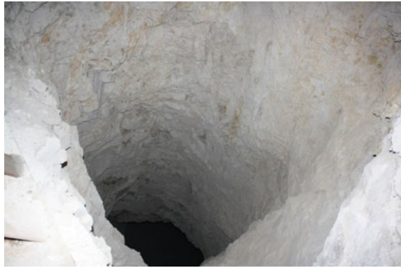
Fig. 1.3 Roughness of mine stope walls
