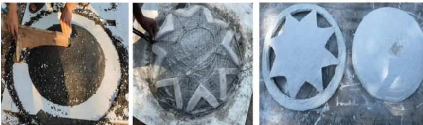
Fig. 13 Casting of conventional and bio-mimicked shell with ferrocement
