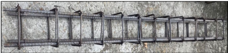
Fig. 4 Reinforcement of beam
