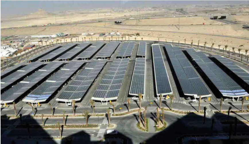
Fig. 1 Saudi Aramco's solar car park in Dhahran
