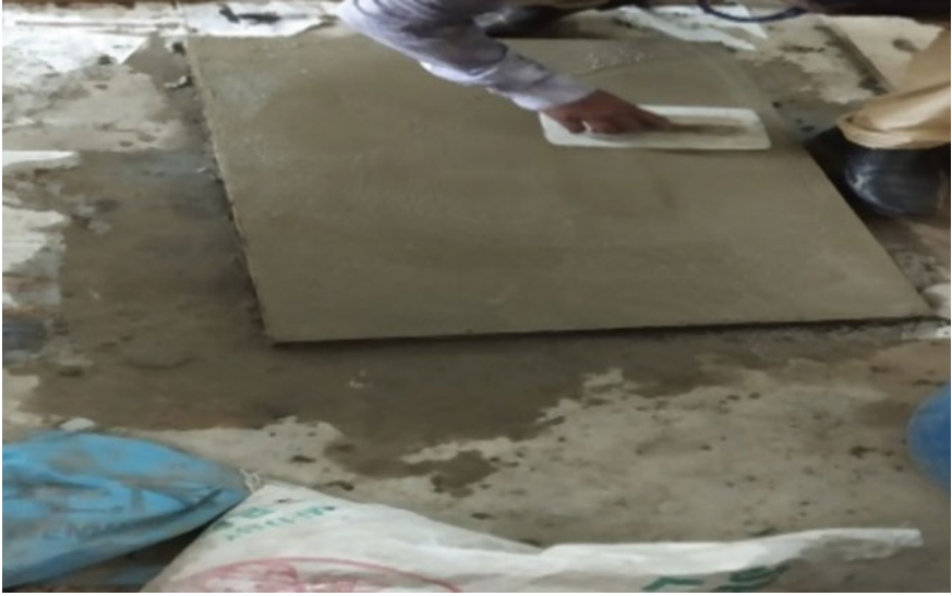
Fig. 4 Wooden bull float application
