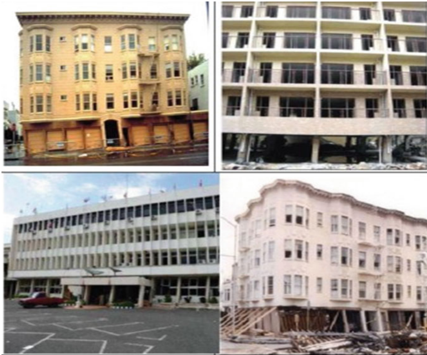
Fig. 1 Buildings failure due to soft storey
