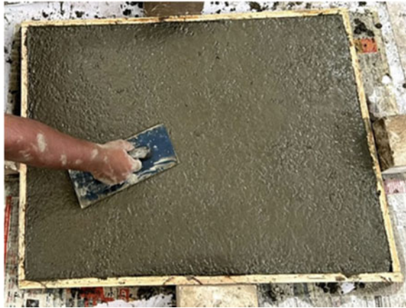
Fig. 4 Bull float application
