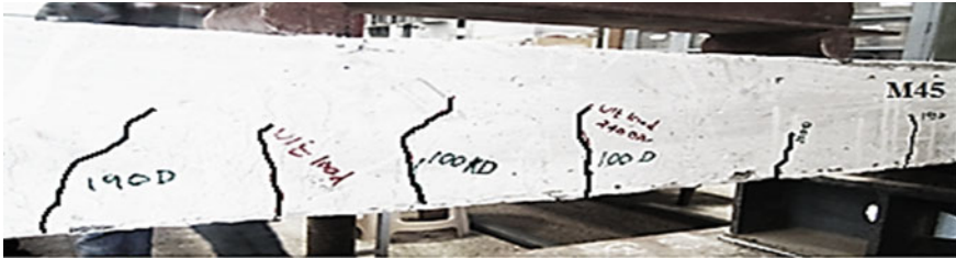
Fig. 6 Typical crack pattern
