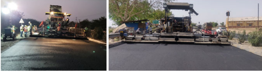
Fig. 6 Bitumen-Friendly Polymer on expressway in India
