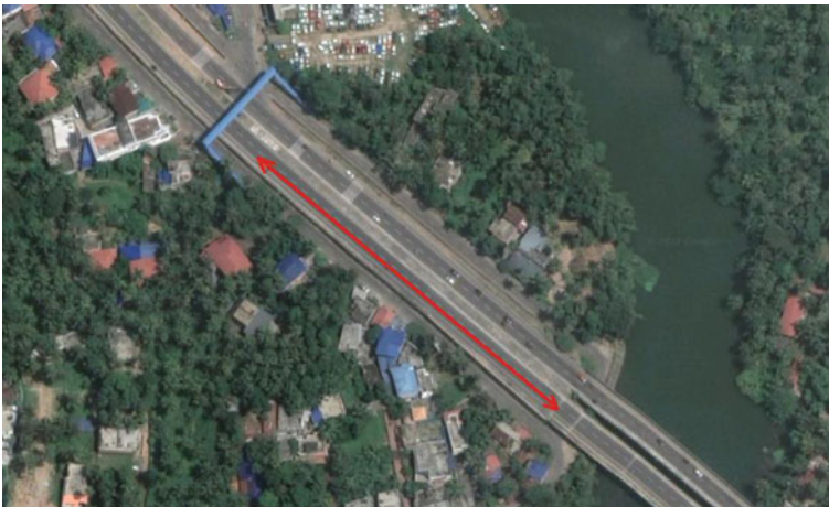
Fig. 1 Aerial view of the NH bypass near Thiruvallam, Thiruvananthapuram
