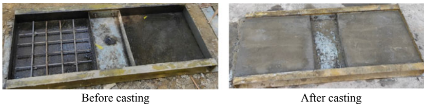
Fig. 1 Casting of concrete panels
