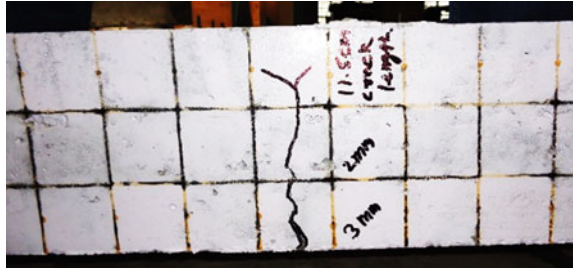
Fig. 14 Cracking in beam A3
