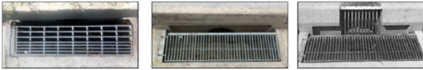
Fig. 4 Three grate inlets with longitudinal bars, transversal bars and transversal bars extended over kerb opening [22]
