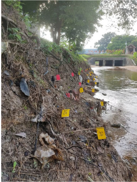
Fig. 3 Erosion pins installed at the riverbank
