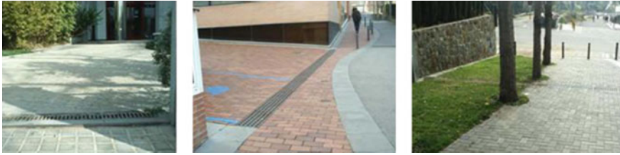
Fig. 5 Typical continuous transverse grates [19]
