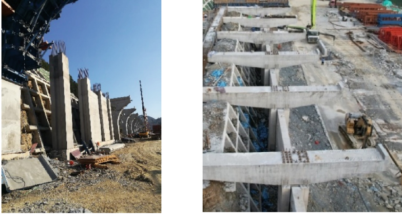
Fig. 2. Prefabricated cantilever composite subgrade structure.
