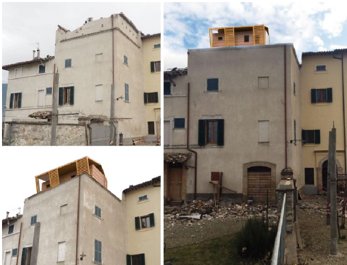
Fig. 7. Intervention of densification of the built-up area by placing the local temporary building organism in place of the roof of an existing building. Existing building before intervention (top left), densification intervention with the temporary module (bottom left and right).
