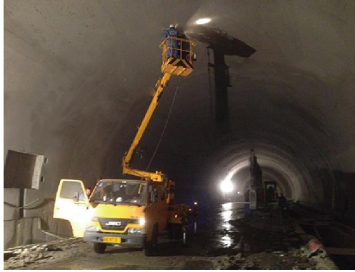
Fig. 7. Radar scan of tunnel vault.
