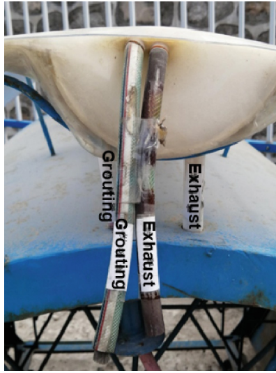
Fig. 5. Tunnel lining grouting simple mold.
