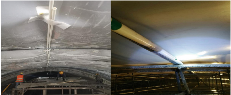
Fig. 4. Photo of embedded pipe fixation in tunnel vault.
