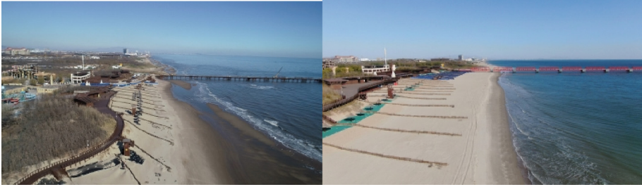
Fig. 3. A figure shows the status of the beach renovation of Beidaihe Dapu River to Xinkai River mouth section. The left is before and the right is after the renovation and restoration.
