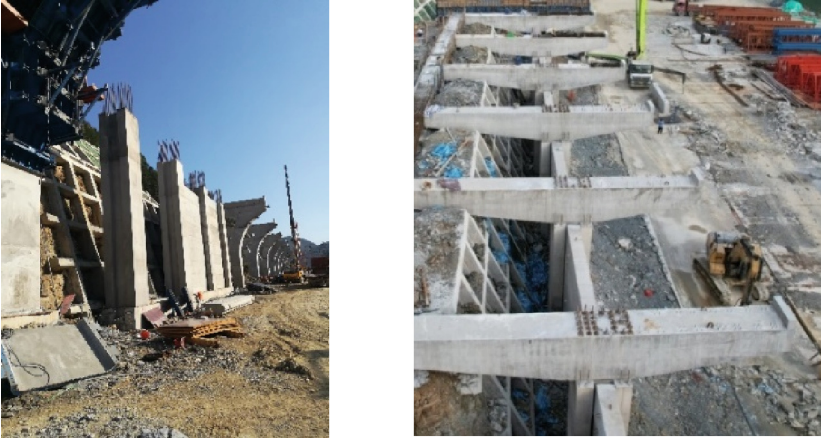
Fig. 2. Prefabricated cantilever composite subgrade structure.
