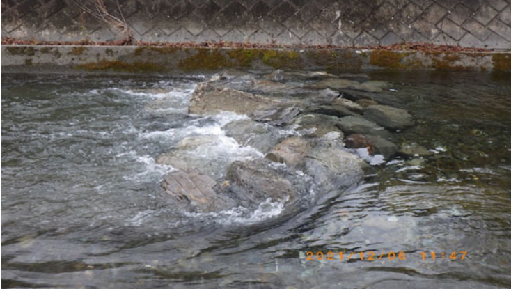
Fig. 22.4 Flow condition around the three continuous rows of assembled boulders
