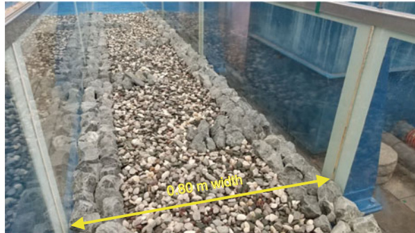
Fig. 22.1 Installation of consecutively assembled boulders in Case 2
