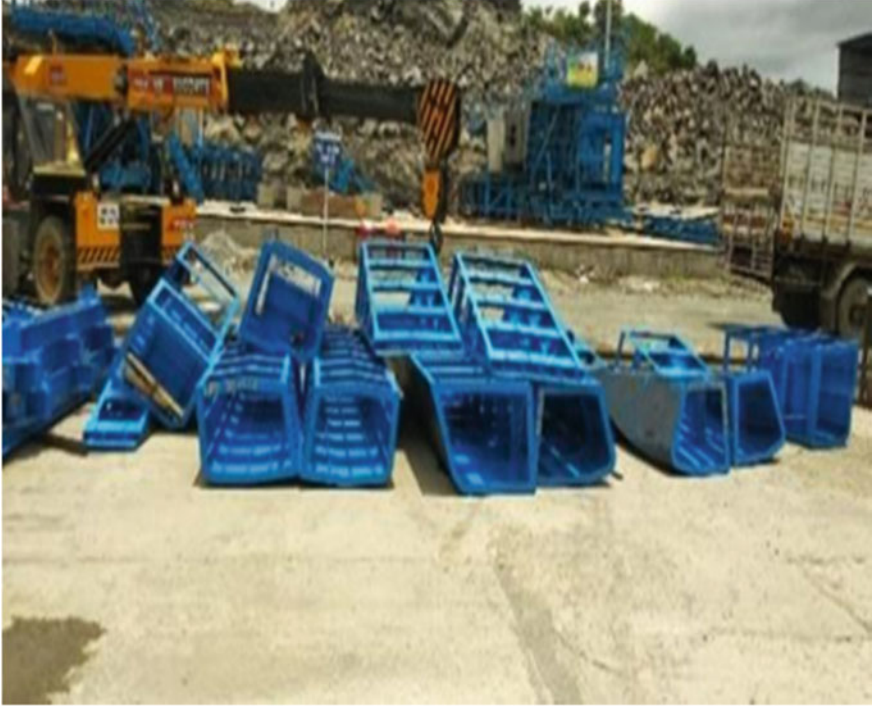
Fig. 2 Panel shifting between bays
