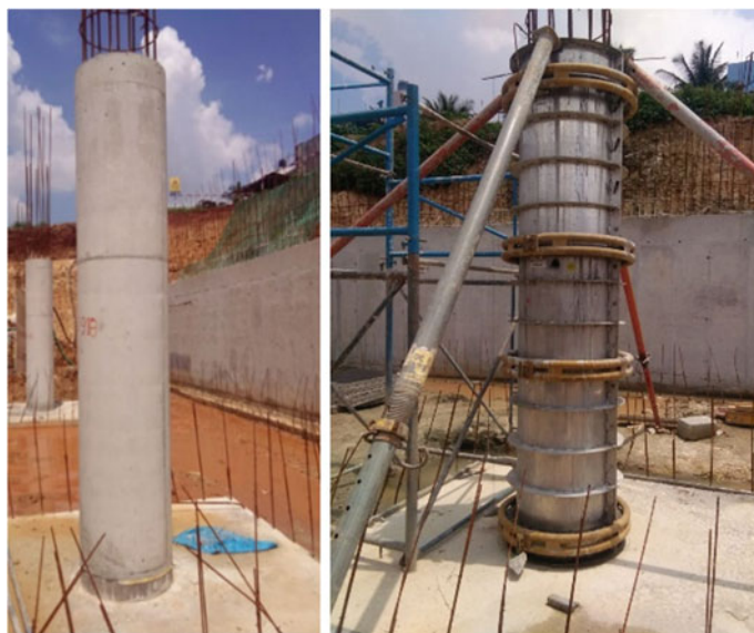
Fig. 3 Circular columns with aluminium formwork
