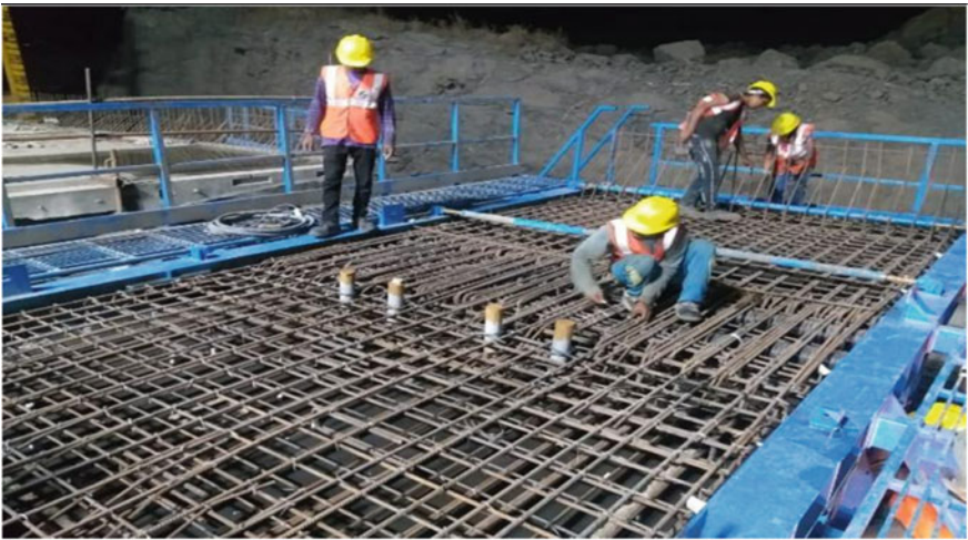
Fig. 3 Tying blister portion on a bed
