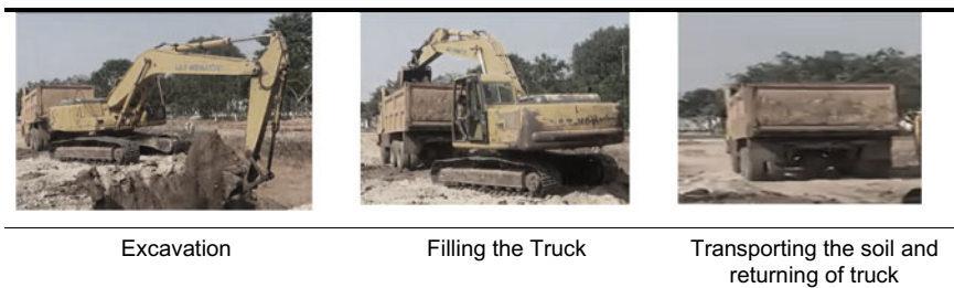
Fig. 1 Process for the mechanised method of excavation
