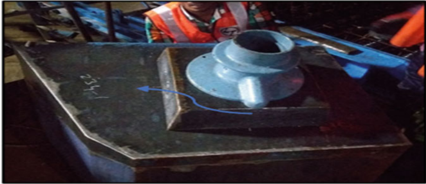
Fig. 4 Wrongly fixed panels
