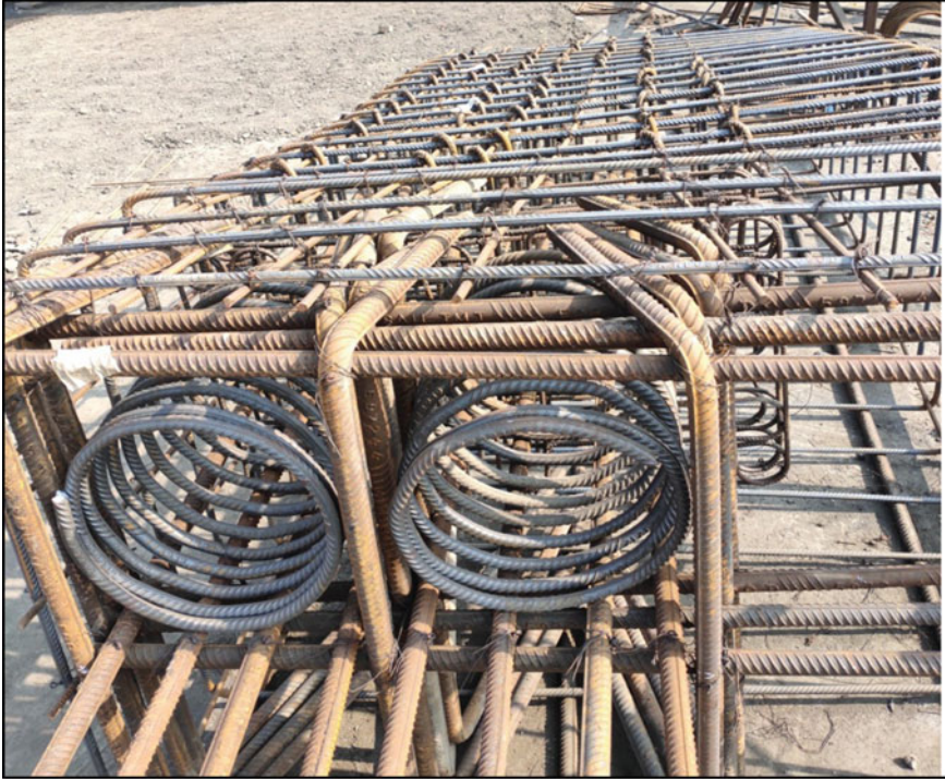
Fig. 10 Segment blister reinforcement mock-up
