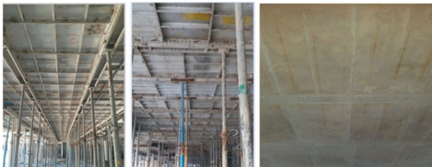
Fig. 2 NTA slabs with aluminium formwork
