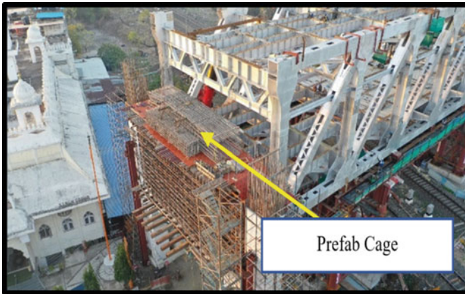
Fig. 15 Prefabricated cage for portal
