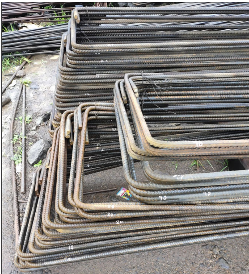
Fig. 11 Numbering of segment web rings
