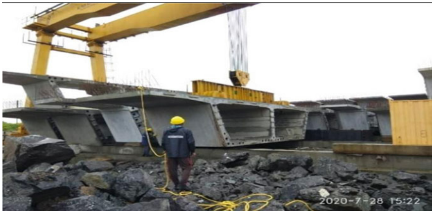
Fig. 7 Segments stacked at SY
