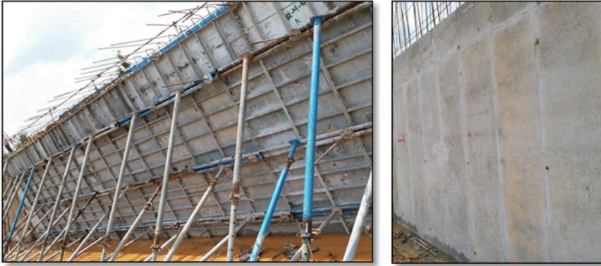
Fig. 1 Retaining wall with aluminium formwork
