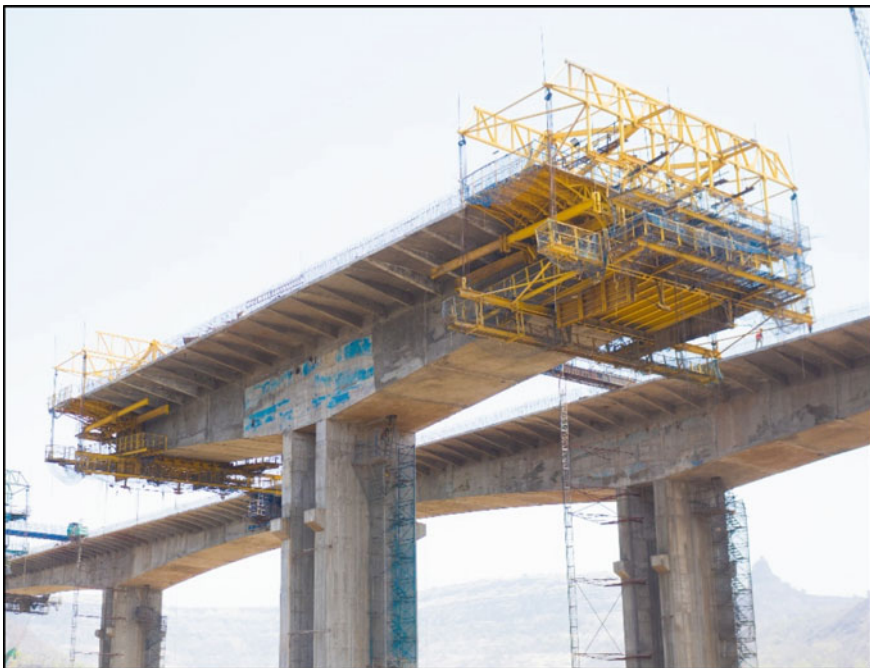
Fig. 4 Segment casting by CFT on either side of pier
