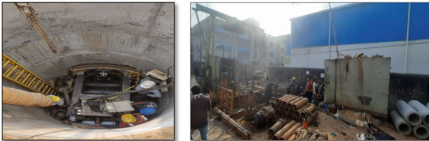
Fig. 2 PTMT job site (Source Cuttack waste water network project, L&T)
