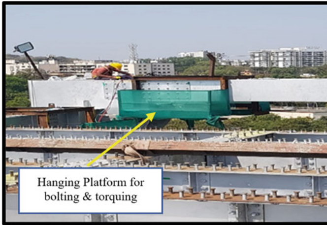
Fig. 11 Typical hanging platform
