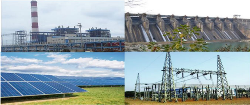
Fig. 7.7 (top to bottom, left to right) 2 × 500 MW TPP for NTPL, solar power generation for BPSCL and NMDC, FGD projects for TANGEDCO, RLA of HYDEL power for DVC, OHPC, TANGEDCO and APGENCO, DDUGJY and IPDS projects for Govt. of Jharkhand and Odisha
