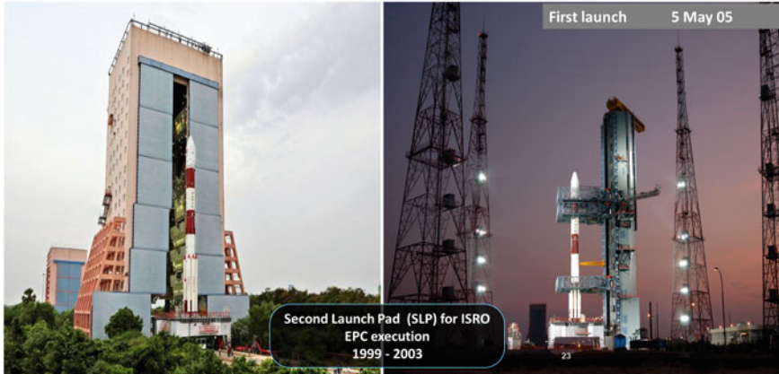
Fig. 7.4 The second launch pad project executed for ISRO
