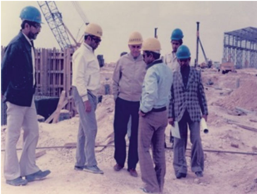
Fig. 5.3 DASTUR engineers at Misurata site
