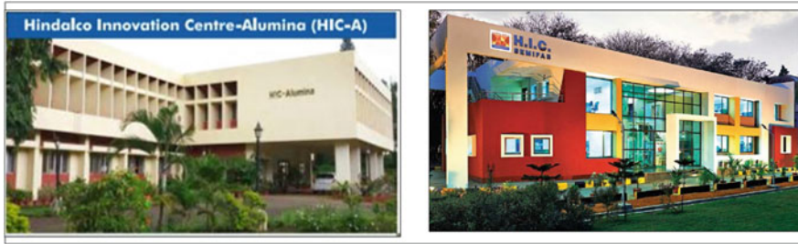
Fig. 6.6 Hindalco Innovation Centre—Alumina and SemiFab
