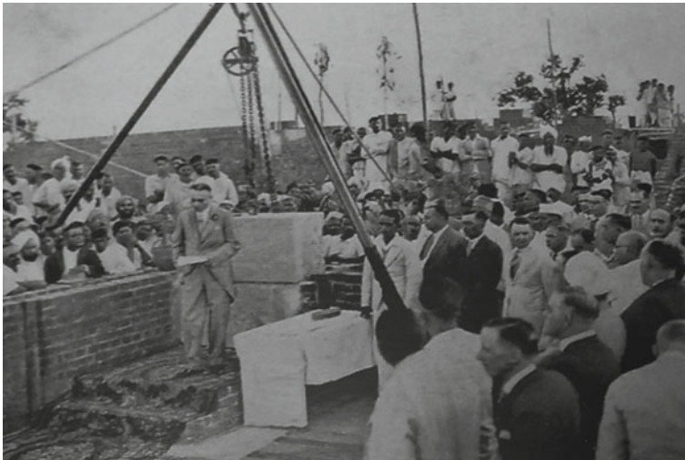
Fig. 1.3 Mr A R Dalal (Director of Tata Sons) delivering his speech during the laying of the foundation stone for the R&D building
