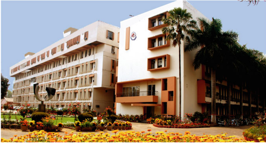
Fig. 7.1 MECON Limited headquarters at Ranchi, Jharkhand
