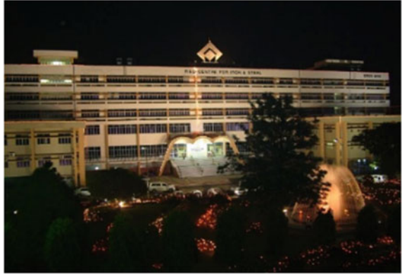
Fig. 18.1 View of the main administrative building of RDCIS, SAIL
