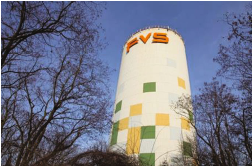
Picture 11.5 Heat storage of Iqony in the “Saar”-region
