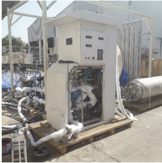
Fig. 3 Test at site with liquid nitrogen
