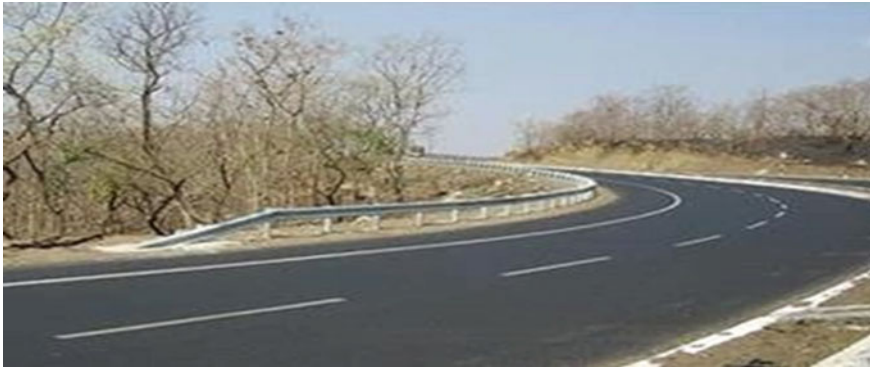
Fig. 13.1 Shows an image of a flexible pavement ( https://civiljungle.com/difference-between-flexible-pavement-rigid-pavement/ )
