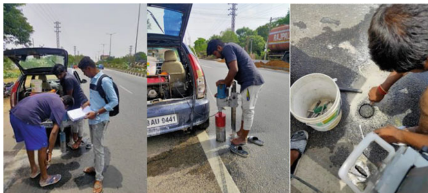
Fig. 8 Core samples collection on the existing pavement, NH-44
