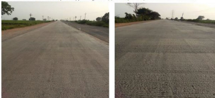
Fig. 2 Present road condition after capacity augmentation (Road Marking yet to be completed)
