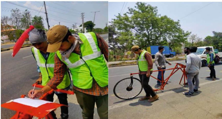
Fig. 3 Roughness survey carried out at the study location
