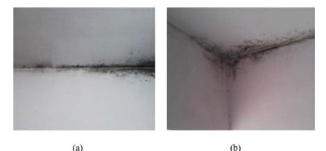
Fig. 2 Mold growth on the internal corner zones of the walls: at the intersection of the exterior wall with the crossbar  $\mathbf{a}$ ; at the intersection of two exterior walls between themselves and at their intersection with crossbars  $\mathbf{b}$
