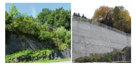
Fig. 14 The 45 years old retaining wall before and after modest rehabilitation
