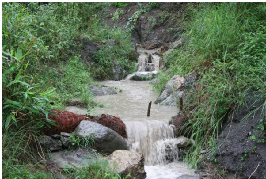
Fig. 1 Check dams of pine needles [5]
