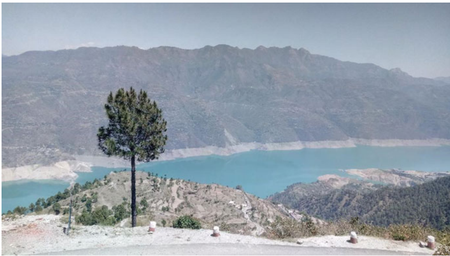
Fig. 5.3 Part of Tehri Dam Reservoir as seen from the Chamba-Chinyalisaur Road in Uttarakhand Himalayas, India
