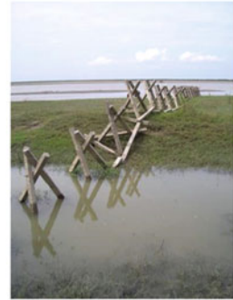
c. Porcupines to Protect River Bank Erosion
