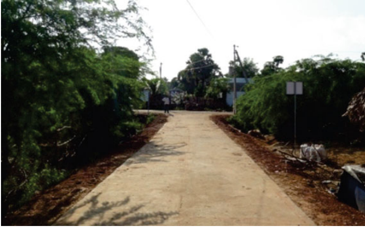
Fig. 7.6 Approach Road in West Godavari District Bridge (Source: NDMA Annual report, 2018–19)
