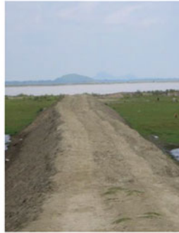
b. Construction of Land Spur
