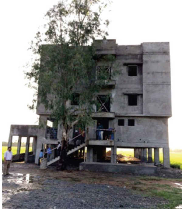
Fig. 7.9 Multipurpose cyclone shelter in Gujrat
