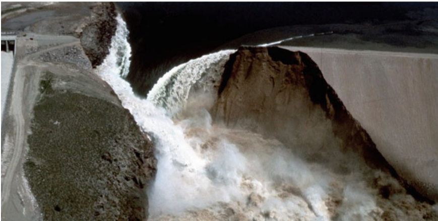
Fig. 1 Photograph of Teton Dam failure [11]
