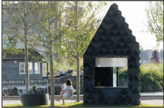
Fig. 4 3D print canal house in Amsterdam [7]
