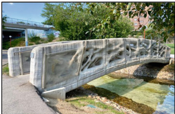
Fig. 2 Castilla-La Mancha Pedestrian bridge [4]
