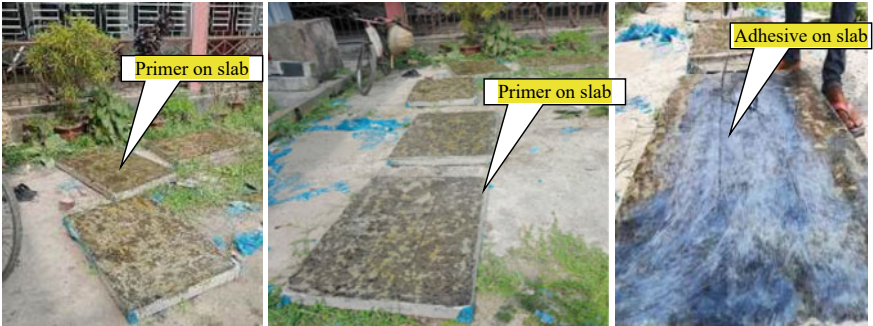
Fig. 5 Applying primer on slab specimen and applying adhesive on slab specimen
