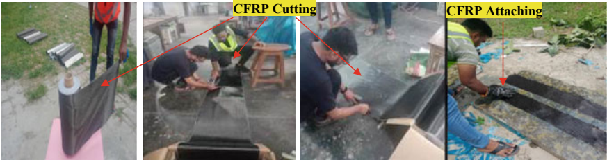
Fig. 6 Cutting and attaching CFRP with adhesive on slab specimen
