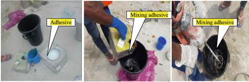
Fig. 4 Mixing primer and base resin and hardener adhesive
