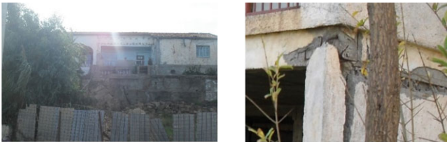
Fig. 1 Disorders caused by the Tizgirt landslide at the level of buildings
