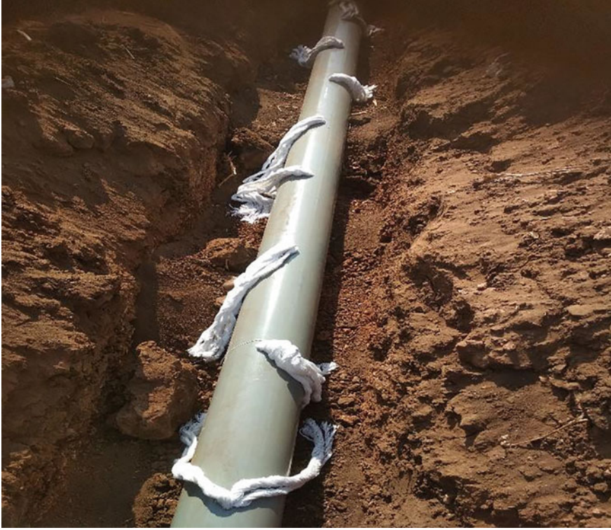
Fig. 4 Wick installation in the pipe on field
