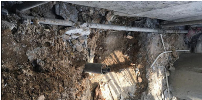
Fig. 22 Capping beam located along the Building A -Building B perimeter wall
