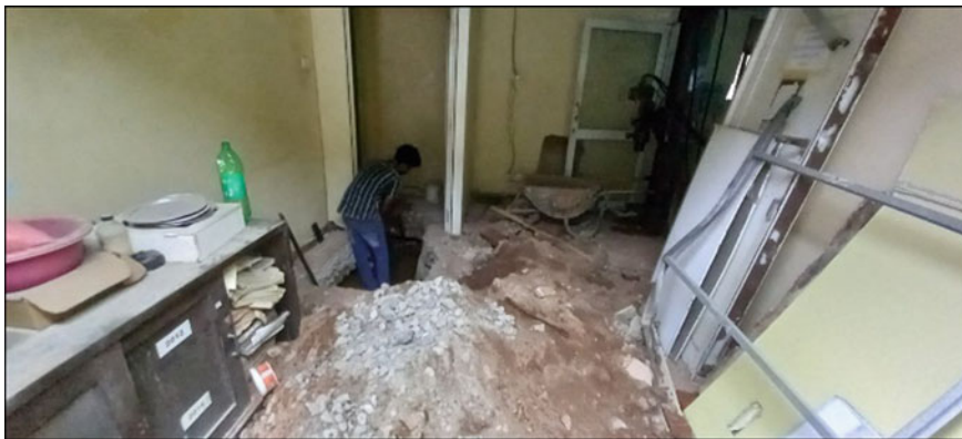
Fig. 7 Exposing column footing
