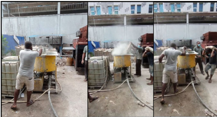
Fig. 11 Mixing of cement grout
