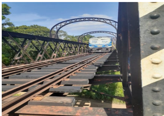
Fig. 1 General view of Kala Oya bridge
