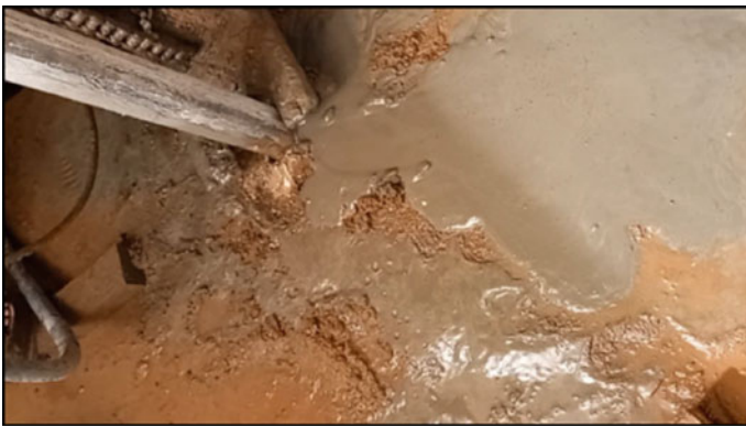
Fig. 15 Grout overflowing from casing while grouting
