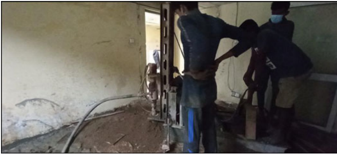
Fig. 10 Drilling of the observation hole
