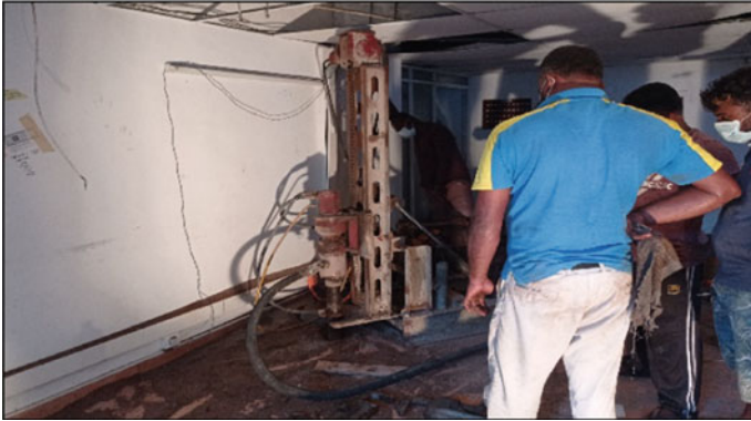
Fig. 14 Grouting of the grout hole
