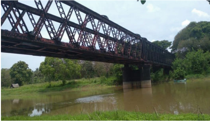
Fig. 2 General view of Malwathu Oya bridge
