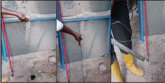
Fig. 16 Checking for traces of grout in observation holes
