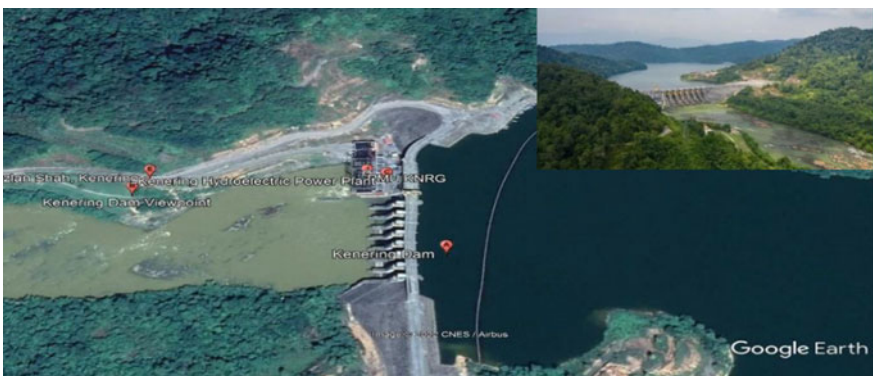
Fig. 4 Kenering Dam in Hulu Perak ( 5.215335^{\circ} 101.097910^{\circ} ) Source Google EarthPro
