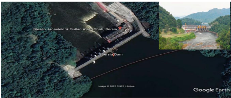
Fig. 3 Bersia Dam in Hulu Perak ( 5.429616^{\circ} 101.208815^{\circ} ) Source Google EarthPro
