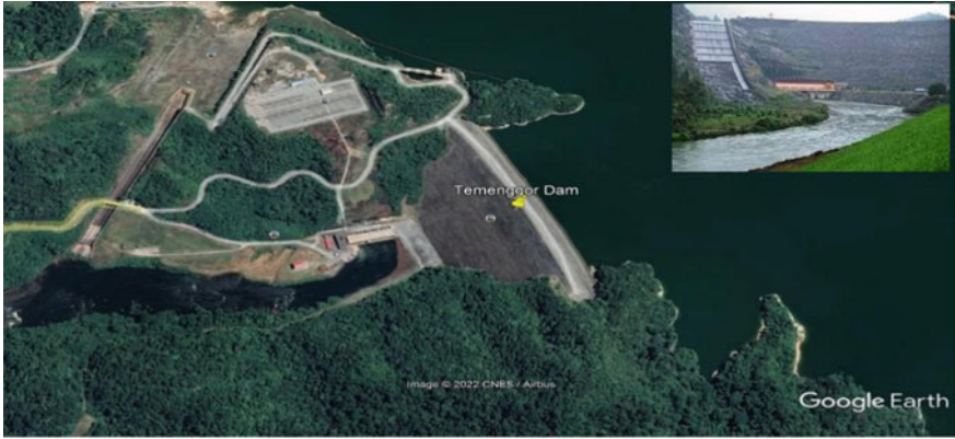
Fig. 2 Temenggor Dam in Hulu Perak ( 5.406234^{\circ} 101.300704^{\circ} ) Source Google EarthPro
