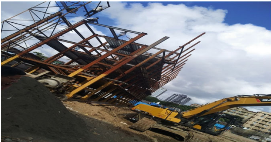
Fig. 11 Actual photo of Prefab work, SRA-Andheri
