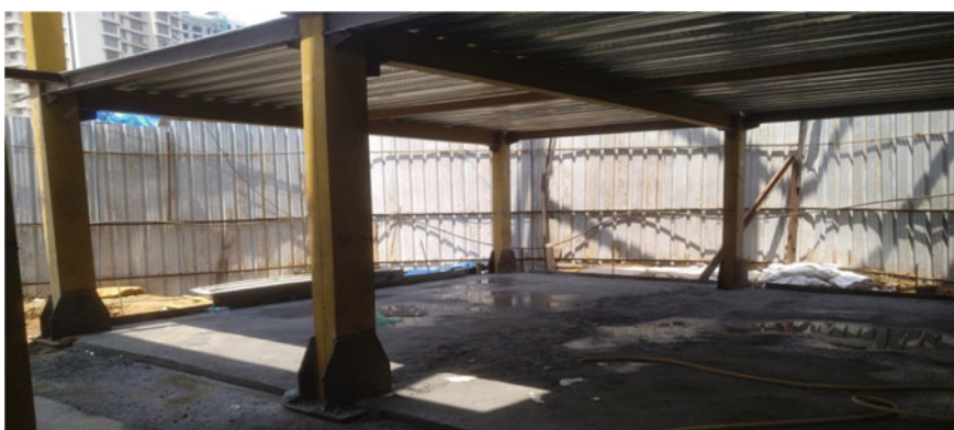
Fig. 13 Actual photo of GF Prefab and channeling work, SRA-Andheri
