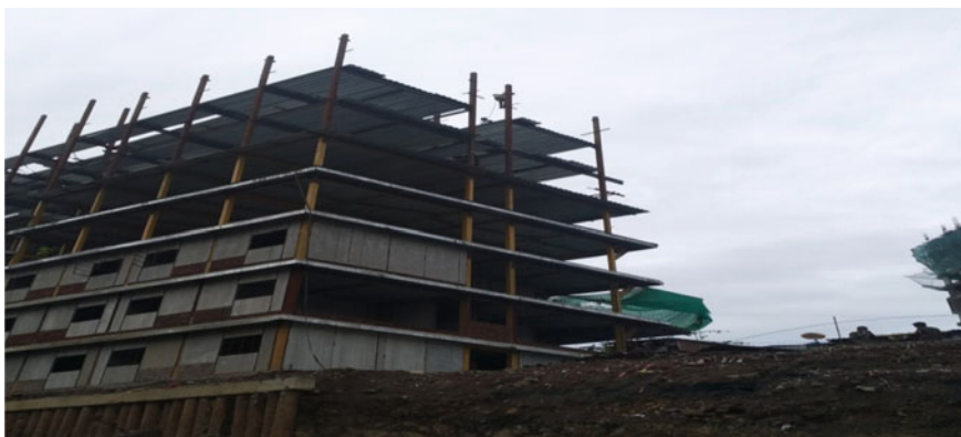
Fig. 12 Actual photo of Prefab and laying of dack sheet, SRA-Andheri
