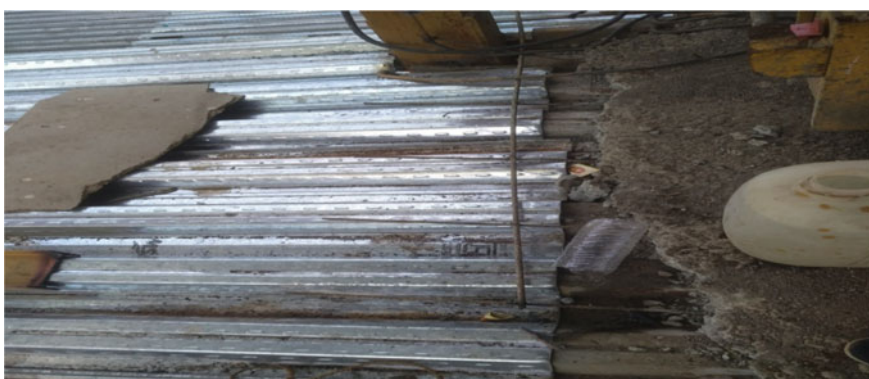
Fig. 14 Actual photo of slab reinforcement work being done, SRA-Andheri
