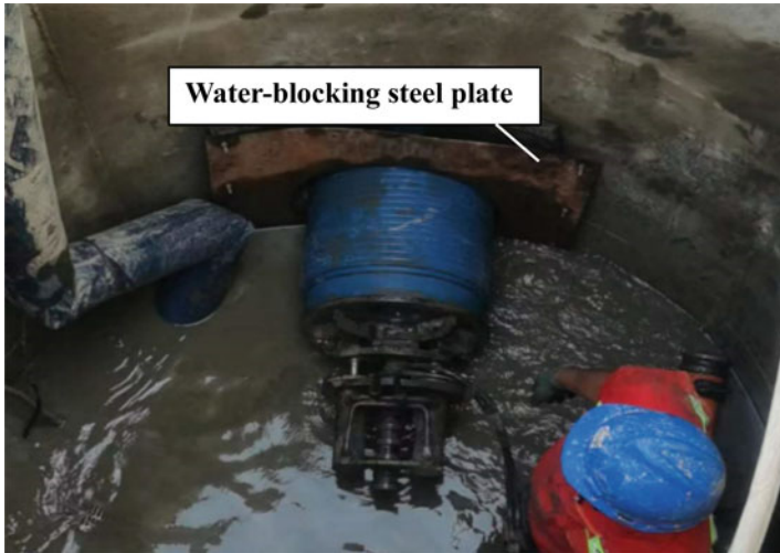
Fig. 3 Schematic diagram of water-blocking steel plate
