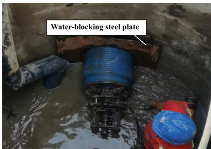
Fig. 3 Schematic diagram of water-blocking steel plate
