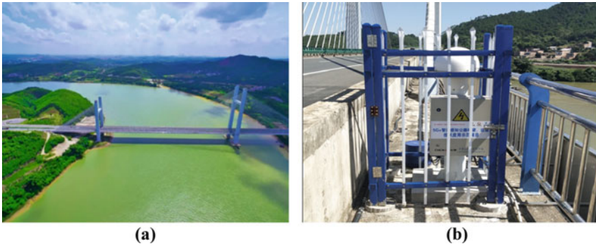
Fig. 1 Monitoring point on Dachongyong (CHC permission)
