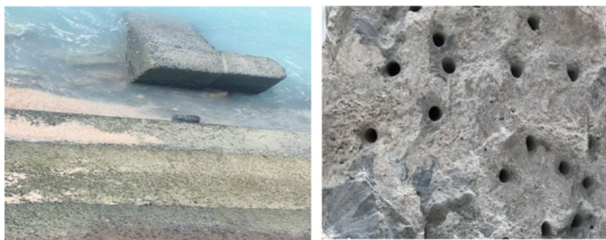
Fig. 1 Example of existing concrete structure (left) and extraction of sample (right)
