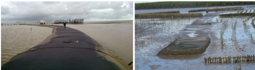
Fig.6 Wave-reducing dike by Geotube in Nha Mat, Bac Lieu (2014)
