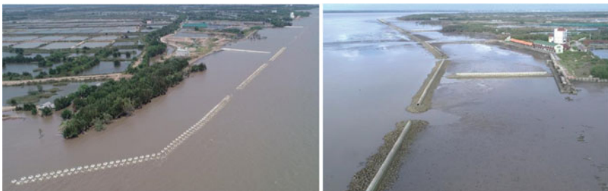
Fig. 29 Detached breakwaters in Con Cong area
