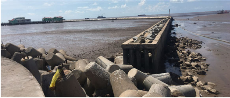
Fig. 17 Spun piles–rock detached breakwater in Nha Mat, Bac Lieu
