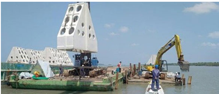
Fig. 21 Installation of BUSADCO Block 1
