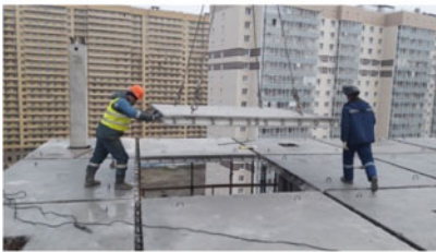
d. Install S-VRO panels
