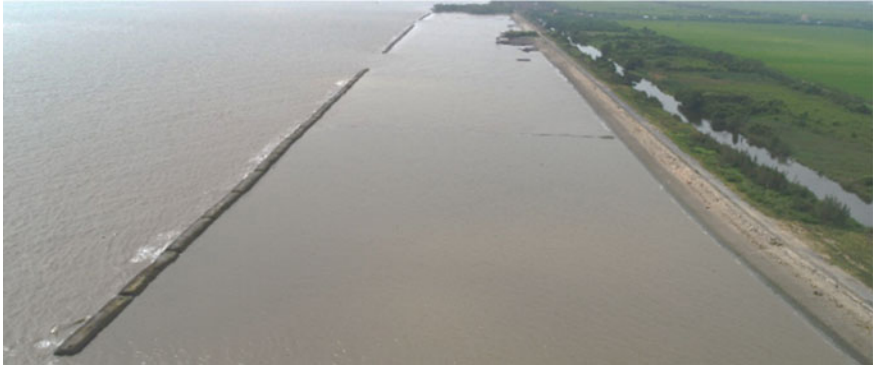
Fig. 8 Geotube breakwater system in Go Cong, Tien Giang
