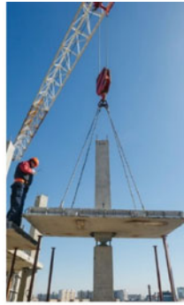
b. Install mushroom panels using cranes
