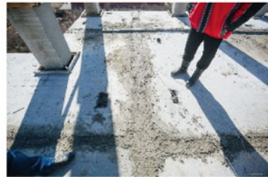
e. Pour concrete into connecting lines
