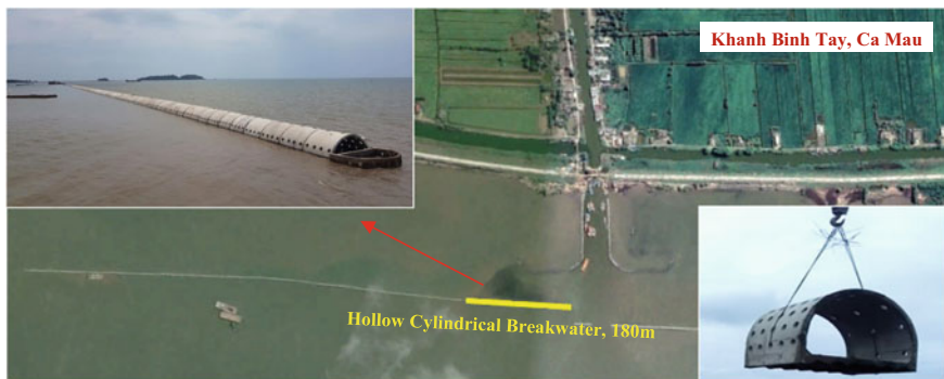
Fig. 19 Pilot modified semicircular breakwater in Khanh Binh Tay, Ca Mau
