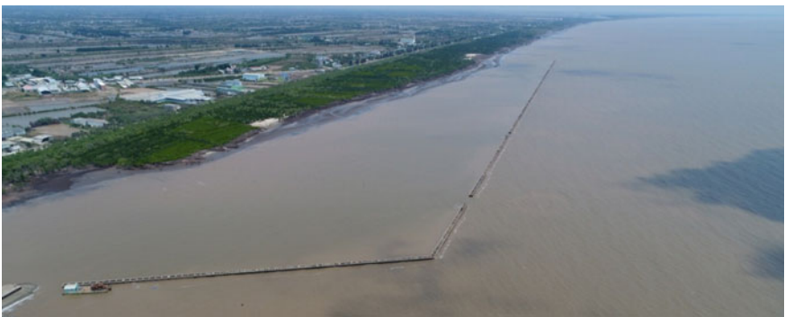
Fig. 16 Spun piles–rock detached breakwater in Ganh Hao, Bac Lieu
