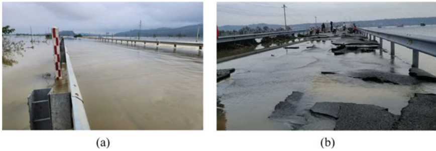
Fig. 1 a Overtopping event on National Highway 1A, Ha-Tinh Province, Vietnam; b Pavement damage due to overtopping event on National Highway 49B, Hue City, Vietnam, October 2020 (Photo from Internet)
