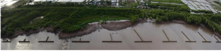
Fig. 3 T-shaped fence with bamboo poles in Bac Lieu province [1]
