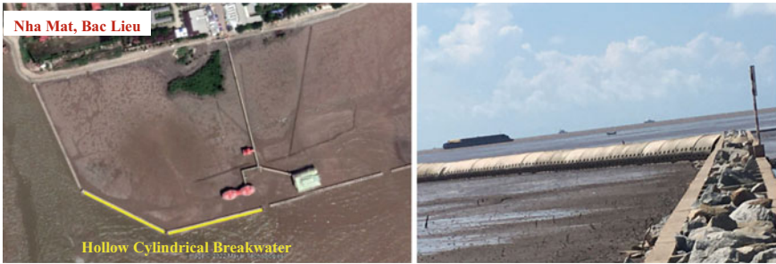
Fig. 20 Modified semicircular breakwater-type DTR304F in Nha Mat, Bac Lieu
