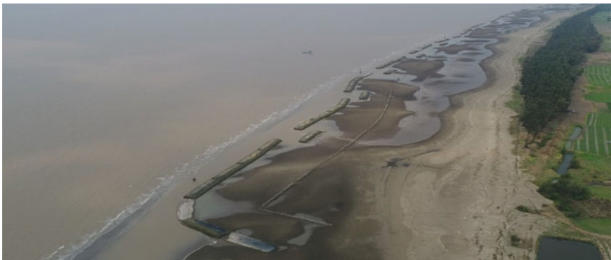
Fig. 9 Geotube breakwater system in Hiep Thanh, Tra Vinh
