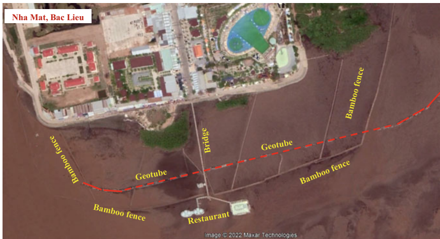
Fig. 5 Layout of the Geotube breakwater line at Nha Mat, Bac Lieu
