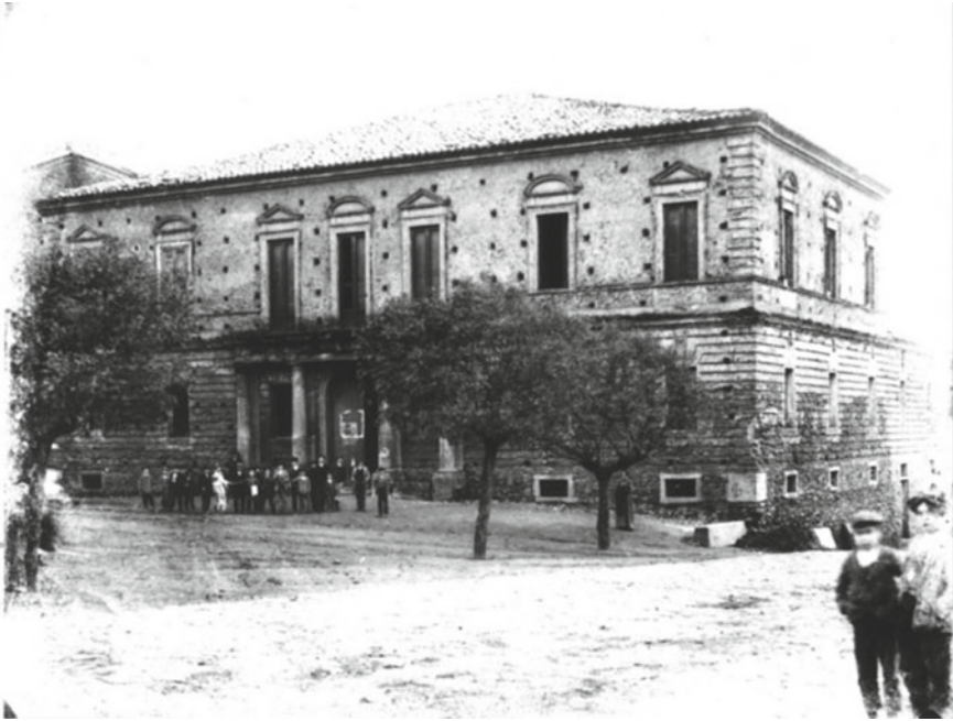
Fig. 11 The “Serrao del Compasso” noble palace is a valid example of a shack-up house still existing in Filadelfia. The building, which is currently in a state of neglect, would deserve an immediate restoration for its architectural and historical value. Source Vito Rondinelli
