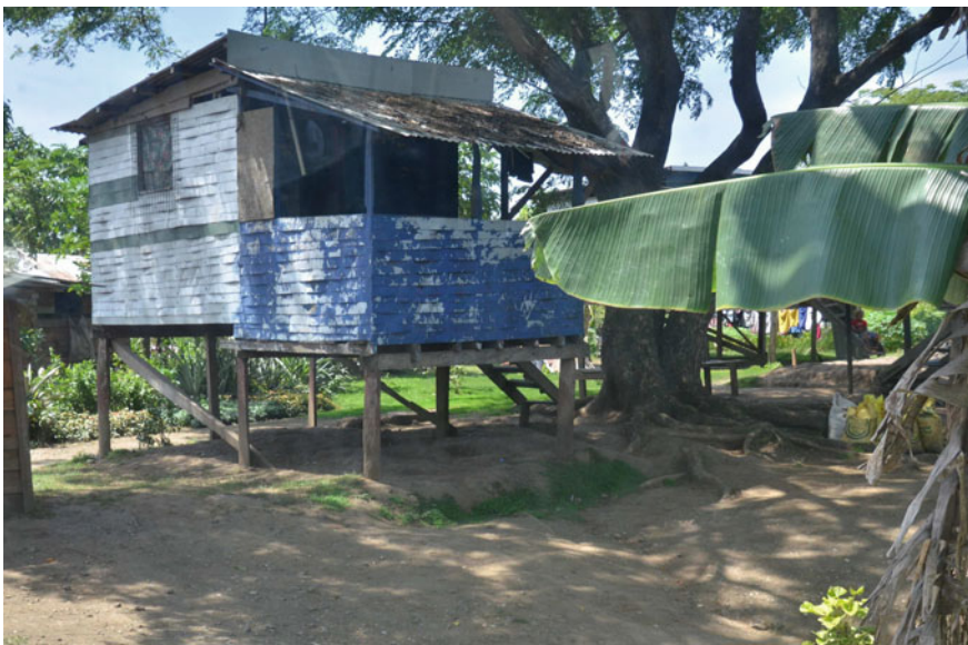
Fig. 6 Bracings used for sturdiness in a house in Honiara (Source Tonkin & Taylor)
