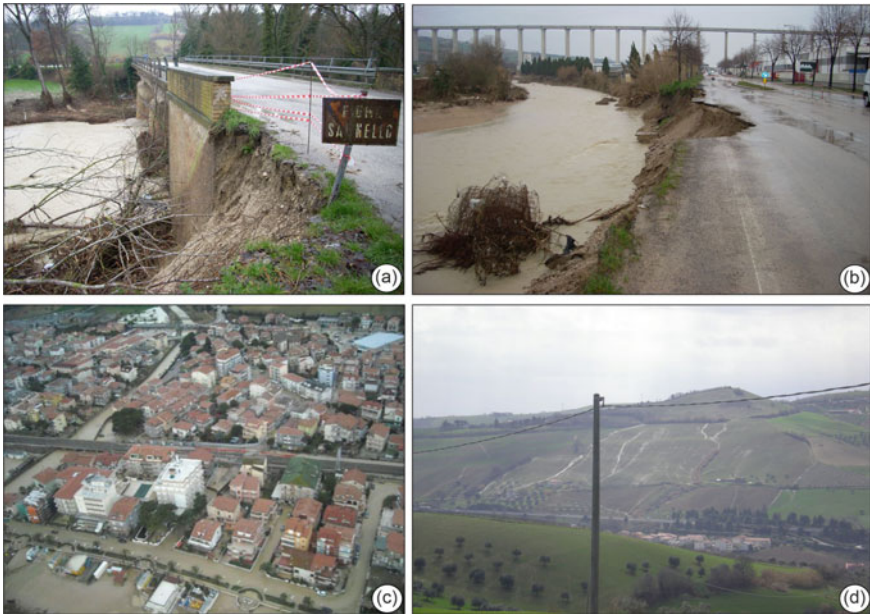
Fig. 12 Flooding and geomorphological effects induced by the 2011 heavy rainfall event. a Salinello River, damage to a bridge; b Salinello River, fluvial erosion scarp affecting the valley road; c flooding phenomena at Pineto, d gully erosion in Pineto hilly area
