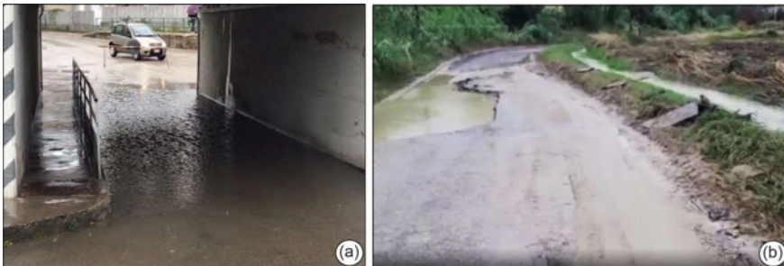
Fig. 18 Flooding and geomorphological effects triggered by the 2018 heavy rainfall event: a underpass flooded and cars stranded in the Pineto area; b detail of damages to roads with rill erosion and mud accumulation (Source www.rete8.it )
