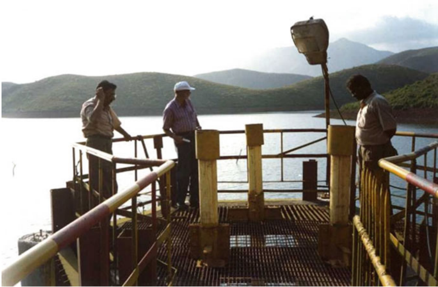
Fig. 10 Aeration pipes in morning glory spillway inlet
