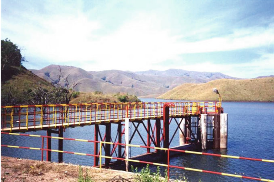
Fig. 8 View of morning glory intake
