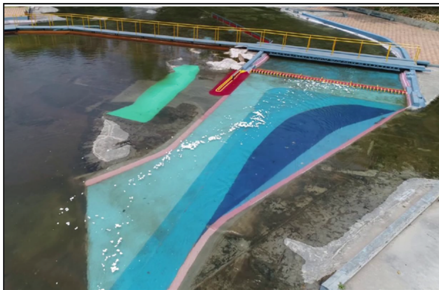
Fig. 10 Flow conditions along the approach channel for PMF condition
