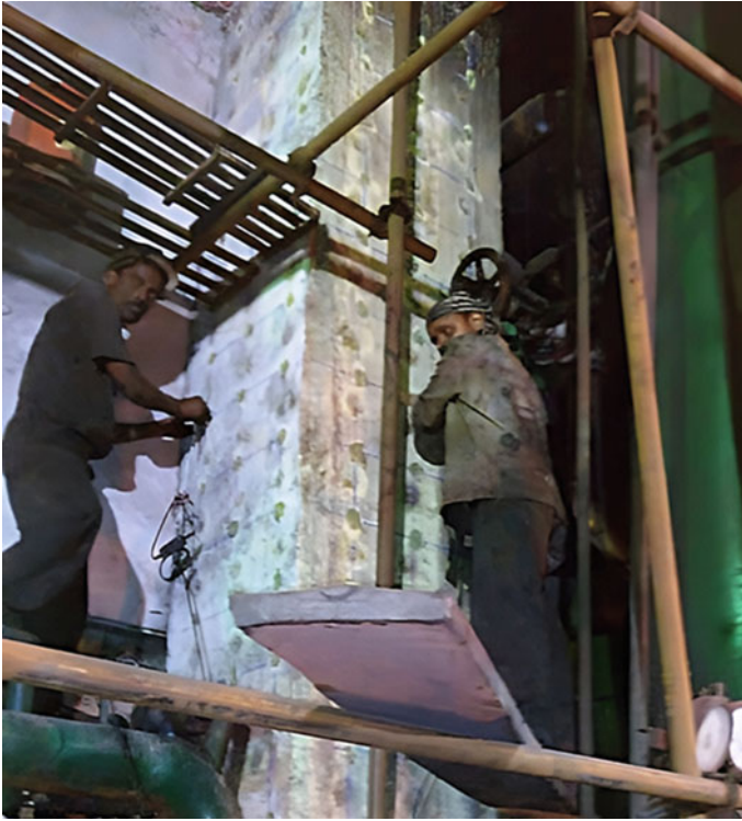
Fig. 2 In-situ ultrasonic test in progress
