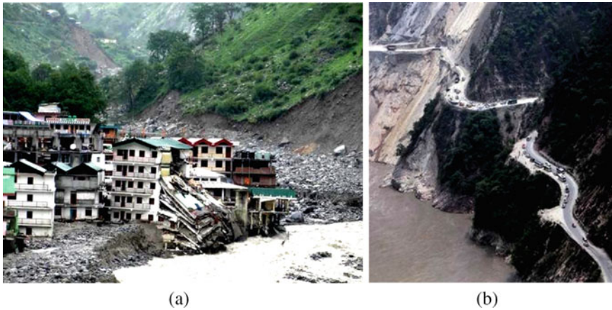
Fig. 2 a Destruction of buildings, b damage of roads [5]
