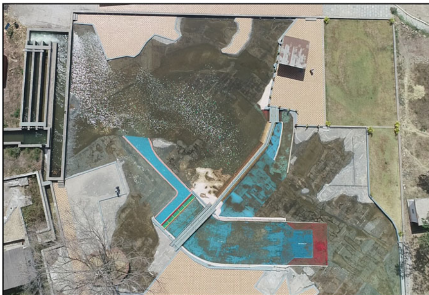
Fig. 5 Aerial view of modified approach channel
