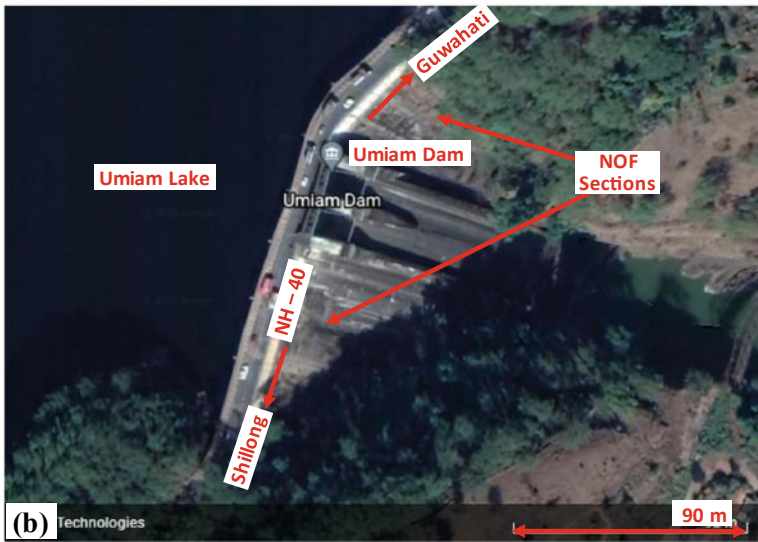
Fig. 1 a Location map of Umiam Dam in East Khasi Hills Dist., Meghalaya. b Downstream view of the dam showing two spillways through three piers and non-overflow sections on either side
