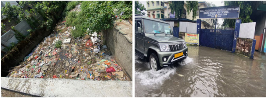
Fig. 4 Canal blockage and flood in Kokrajhar town
