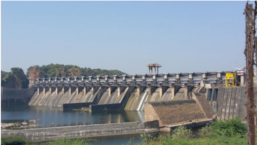
Fig. 3 Downstream view of Kadana Dam, Gujarat
