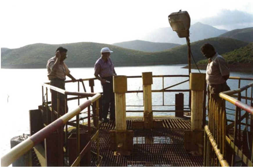
Fig. 10 Aeration pipes in morning glory spillway inlet
