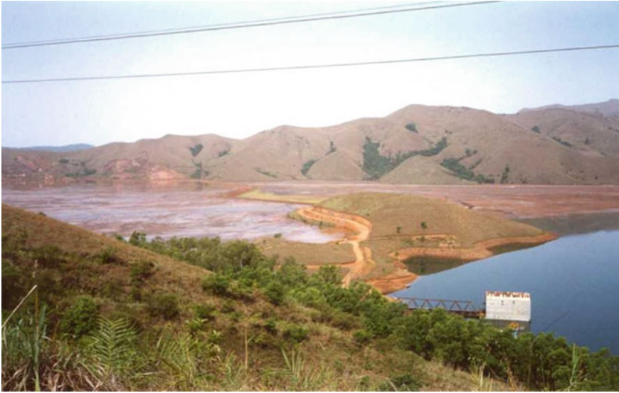
Fig. 5 View of tailing deposit from intake tunnel leading to plant
