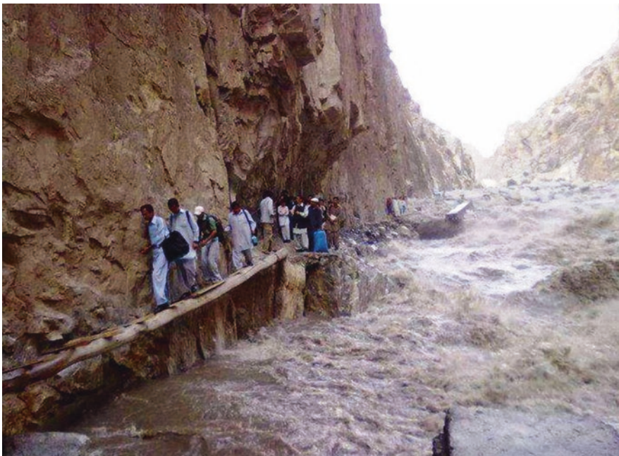
Fig. 8 Infrastructure damage due to flooding
