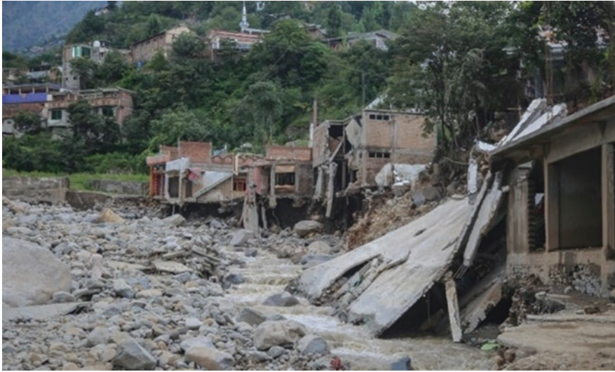
Fig. 6 Damage due to flood
