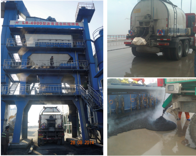
Fig. 7.38 The guss-cooker and paver for gussasphalt
