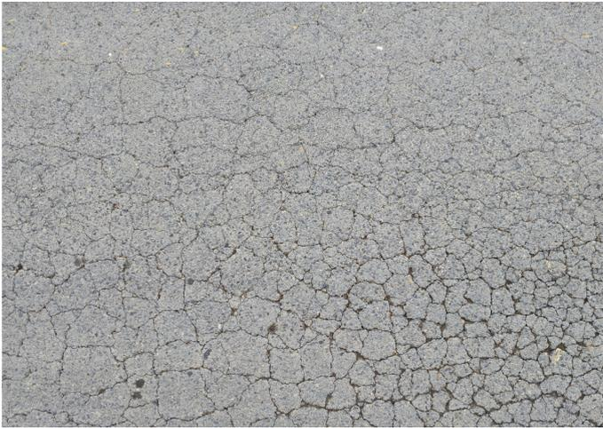
**Fig. 7.21** Fatigue cracking in asphalt pavements
