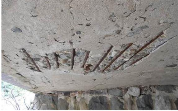
Calcium hydroxide in cement mortar is dissolved by transforming into soluble calcium hydrogen carbonate, leading to the decomposition of other hydrates, and enhancing the corrosion effect.
