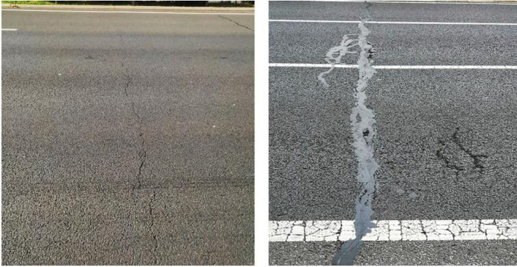
**Fig. 7.19** Thermal cracking on asphalt pavements
